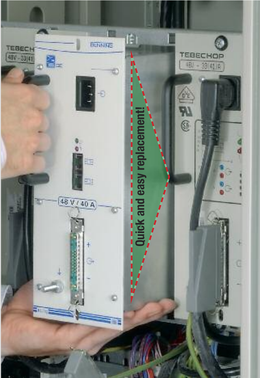
Fig. 5: FIT-FORM-FUNCTION – this means: Simply replace it! System modernization with TEBECHOP SE modules
